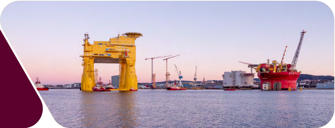
For the first time in history, Aibel has two offshore wind platforms at the Haugesund Yard at the same time.
